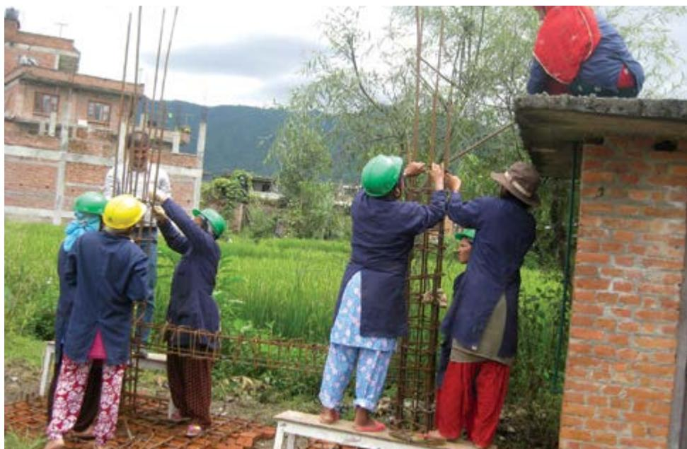
Women in Lamatar placing ties in right way to align the steel bars of pillars to provide additional strength. Photo by: Sudin Pradhan/Oxfam
