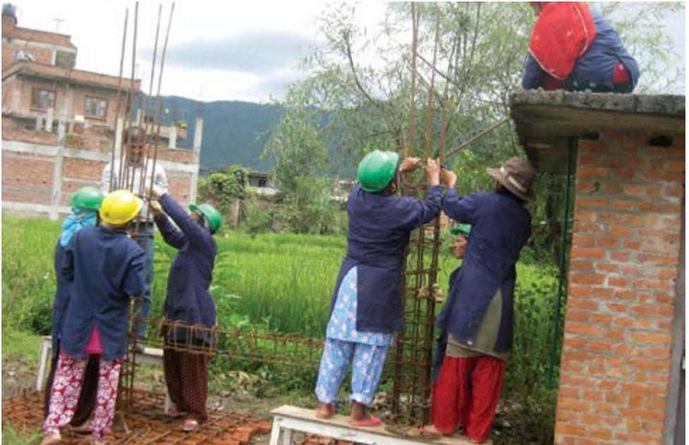
Women in Lamatar placing ties in right way to align the steel bars of pillars to provide additional strength. Photo by: Sudin Pradhan/Oxfam
